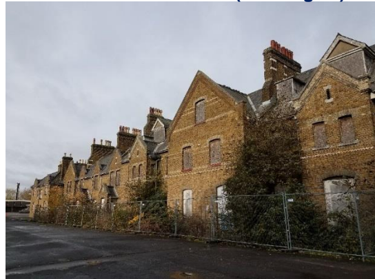
Figure 6.3.7A "Coronation Street" - Fusiliers' Block/Junior Ranks Single Living Accommodation - JRSLA (Building 18)
