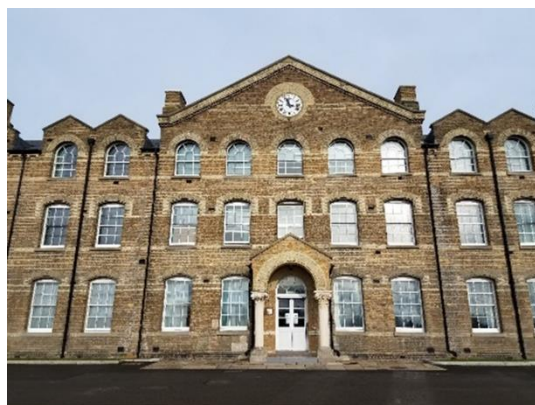
Figure 6.3.6 A Officers' Quarters and Mess (Building 1)
