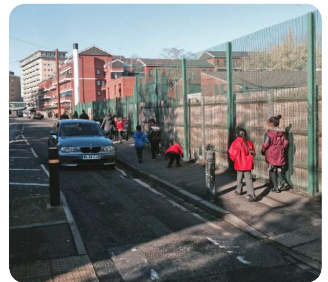
Inadequate narrow footways on Victoria Road
