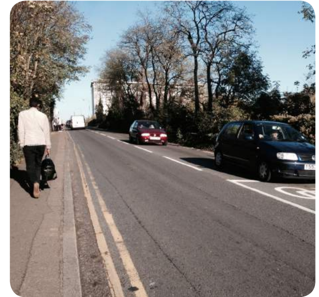
Narrow footway at Hounslow Road bridge
