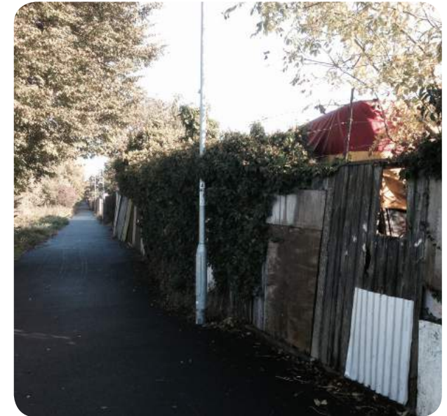
Poor quality connections
