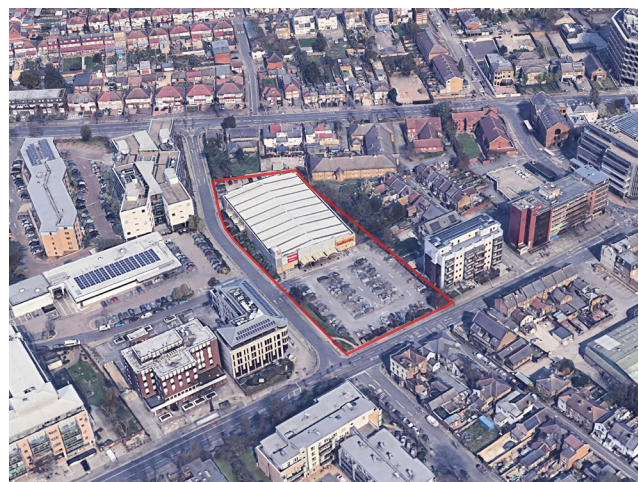
Aerial view of existing area
