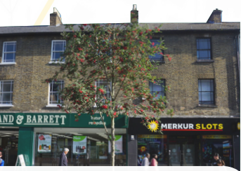
Mid-19th century, tripartite windows, slate roof, and chimney stacks
