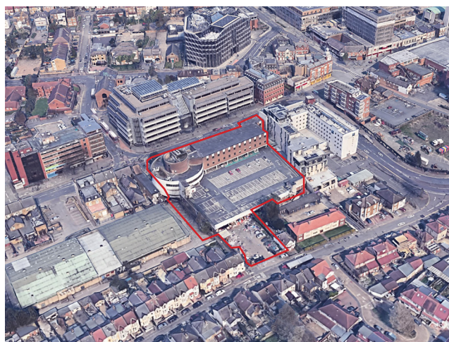
Aerial view of existing area
