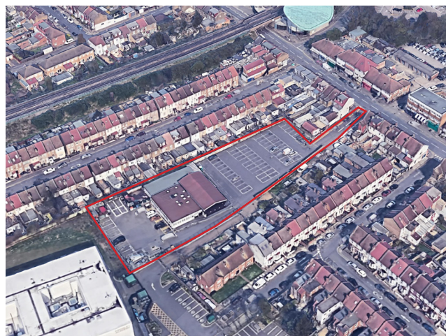
Aerial view of existing area
