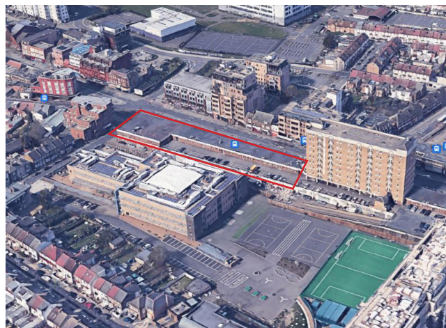
Aerial view of existing area
