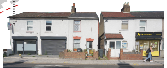
Two storey late 19th century cottage style terraces, mostly retail, and heavily altered - including doors, windows, roofs, and boundary walls.
