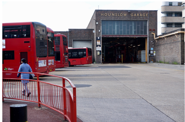
Figure 1.50: Photos of the existing bus garage
