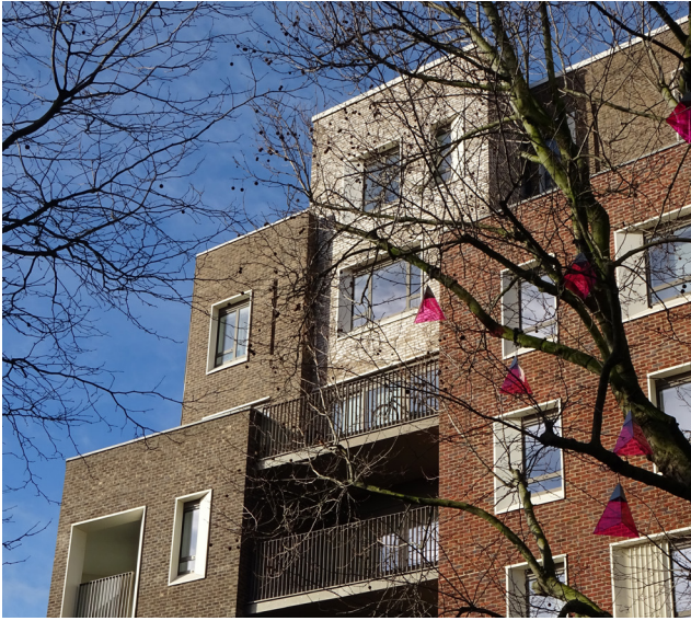
Tarling House, Elephant and Castle, London. Designers unknown. Photo: Allies and Morrison.
