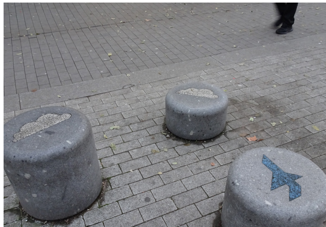
Hounslow town centre lacks greenery which would soften the urban environment and bring greater climate resilience. The grey low bollards are particularly difficult to see, and as such are a barrier to accessibility.
