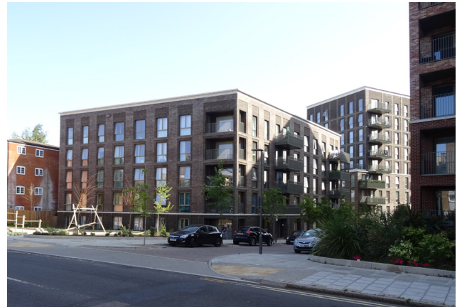
Mediating between the town centre and surrounding suburbs with a 5-11 storey scheme that has strong frontage to the main road. A good example of high density without towers. Precedent example: Lexicon, Harrow © Allies and Morrison
