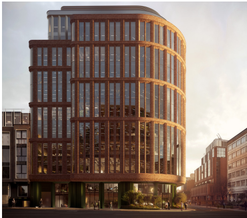
Using double height frames can play with the sense of the number of storeys. Precedent example: Francis Grove © MATT Architecture
