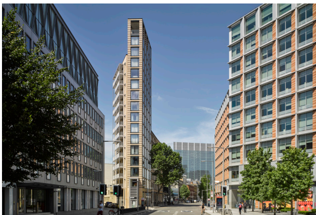
Where sites are smaller, high density can still be achieved using height without its massing feeling intrusive. The block responds to the street layout and acts a local landmark. Precedent example: 67 Southwark Street © Allies and Morrison
