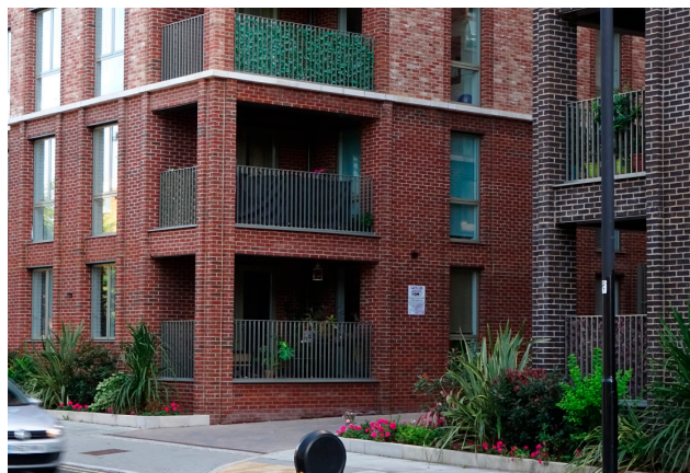
Incorporating well designed landscape and planting, which offers play space and softens the edges with the public realm. Precedent examples: The Lexicon, Harrow © EHW Architects
