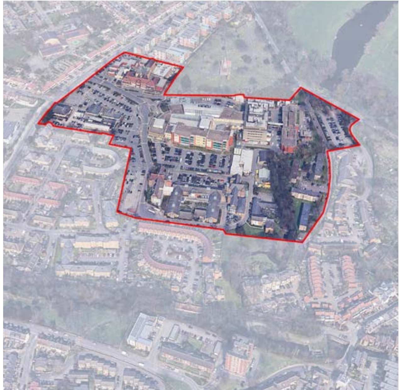
Figure 7.195: West Middlesex Hospital Area of Search - existing aerial
