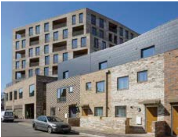
Image 3.2: An eight storey building in an area with a three storey context appears tall
