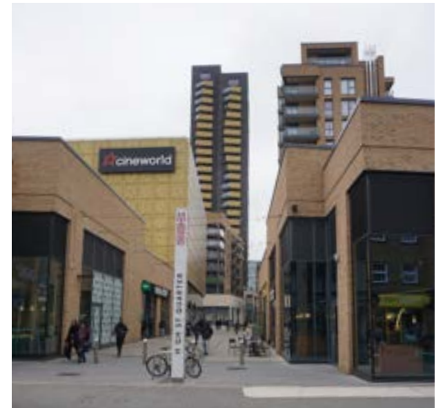
Image 3.4: Recent towers emerging from urban blocks in Hounslow's High Street Quarter
