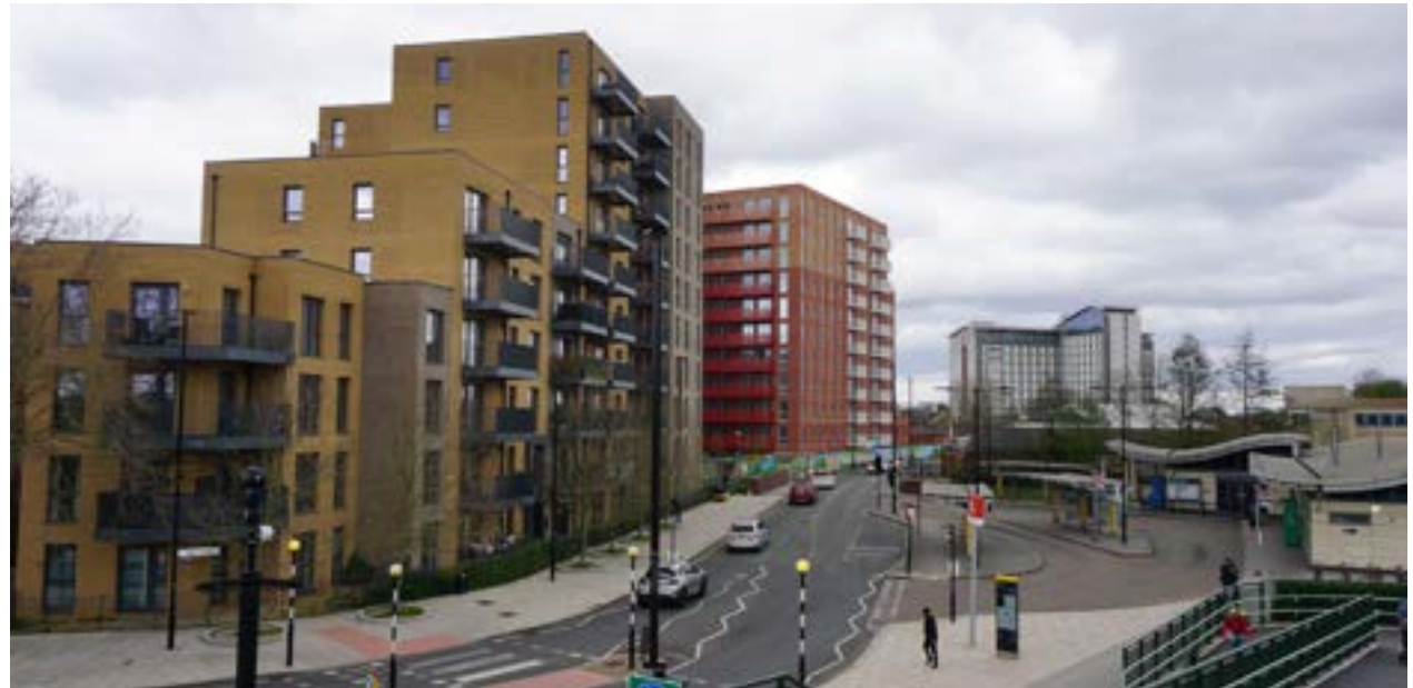
Image 4.5: Tall residential buildings next to Feltham station
