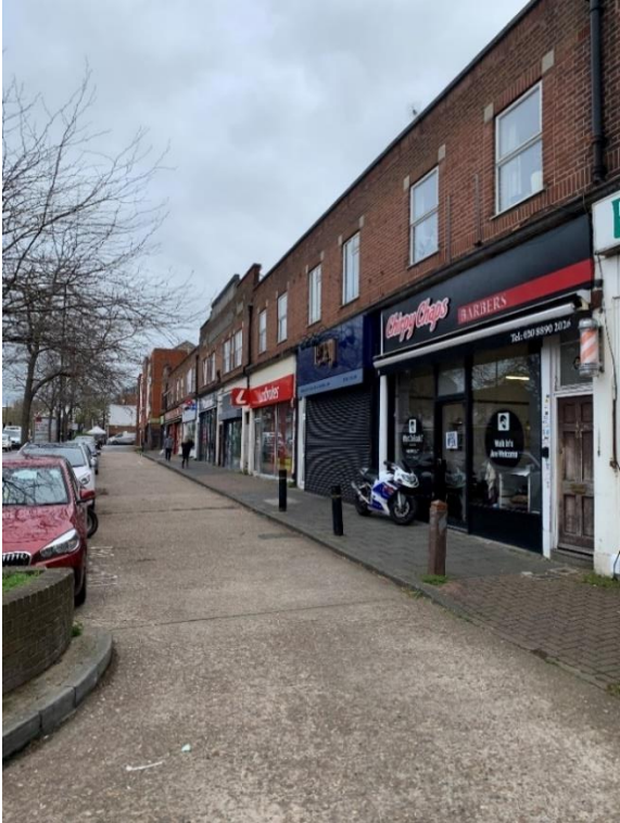
Figure 4.7 – View of the shopping parade at Cavendish Terrace
