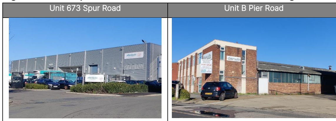
Figure 3.12 Examples of industrial units at North Feltham Trading Est.
