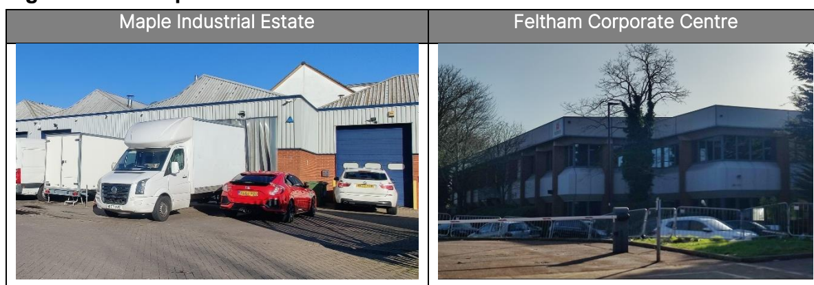
Figure 3.8 Examples of industrial units northwest of Hanworth Park
