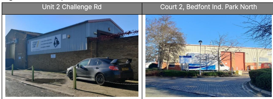
Figure 3.7 Examples of industrial units a Bedfont Industrial Park North
