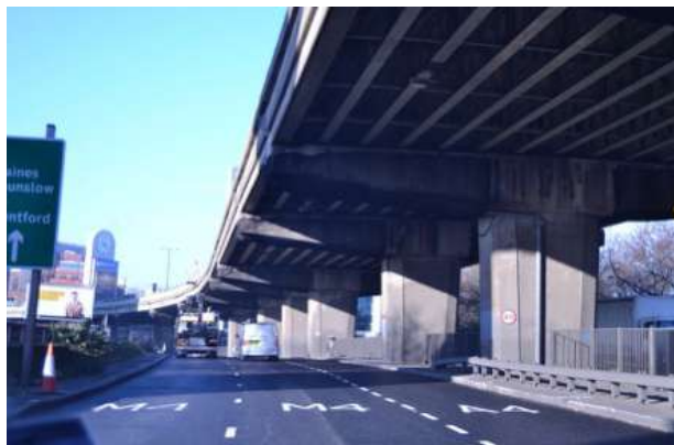
Great West Road below the elevated M4
