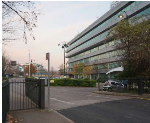
Offices facing onto Great West Road
