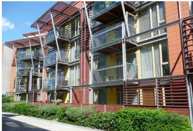
Example of residential development (Millennium Village, Greenwich)
