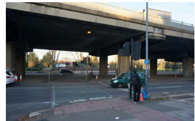
Poor quality walking environment under the M4
