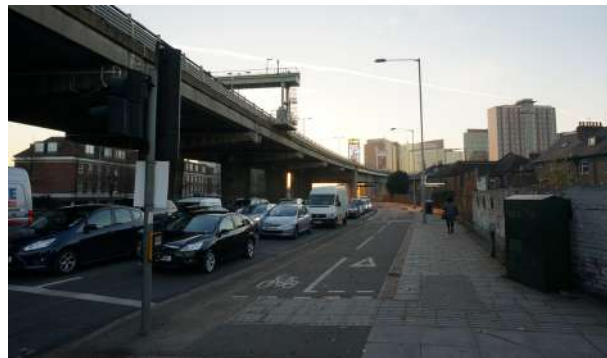
Elevated M4 corridor runs through this area
