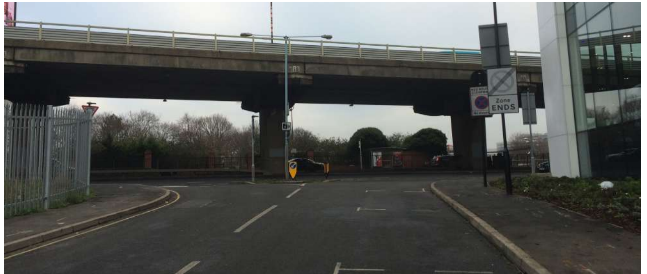
The area suffers from a poor image and lack of connectivity
