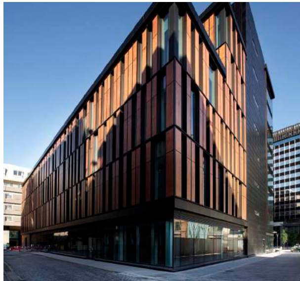
High quality new office buildings
