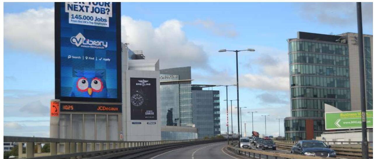
Advertisement panels on the elevated sections of the M4
