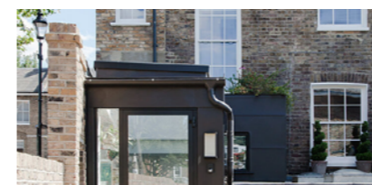
Precedent example: Sensitive extension and refurbishment of existing property enhancing overall energy performance - Barnsbury Road by George & James Architects © Megan Taylor
