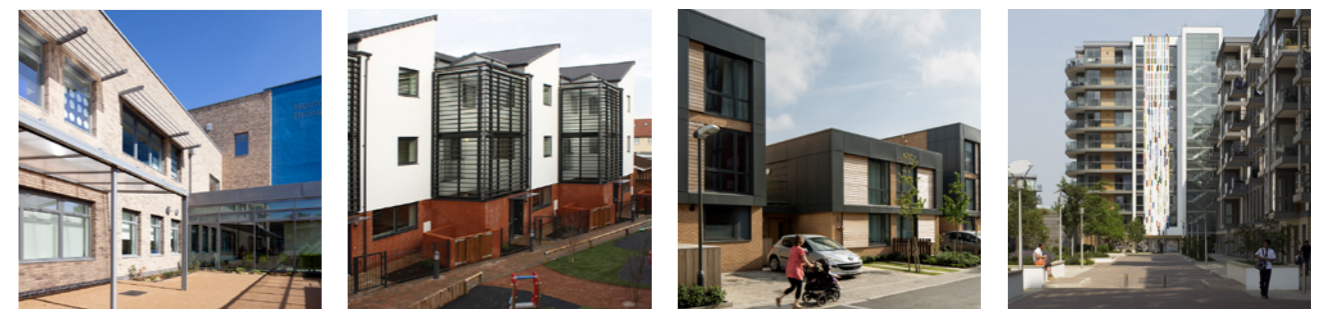
Photos of more recent development across the Borough - many falling within the 'modern urban' category
