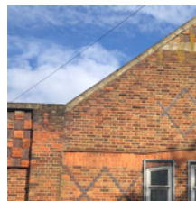
Red brick and detailing
