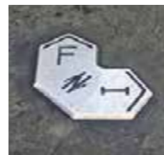
Fig B6.19 Example of town centre signage: Stainless steel plaques embedded into the pavement to indicate the shortest distance between the two train stations in Bradford.
