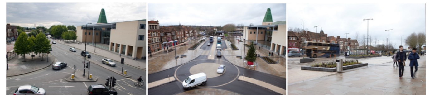
Fig B6.20 Frideswide Square, Oxford (the Urbanists) Before and after. The improvements included removing the multiple lanes of traffic and introducing low curbs, high quality paving, crossing points, a wide central reservation and greenery as traffic calming measures. It signals a welcoming entry to the city's busy station.
