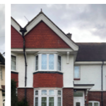
Double height bay windows
