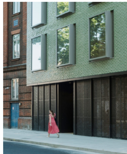
Fig B1.16 Mae-Pegasuslife. This scheme uses green glazed tiles, an example of high quality materials
