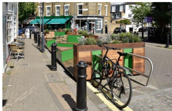
Fig B10.20 Parklet in Hammersmith. Example of an improvement to dead space.
