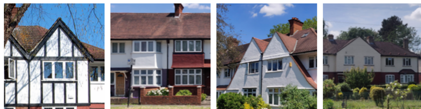
Half-timbering Bay windows Pitched roofs Brick and render
