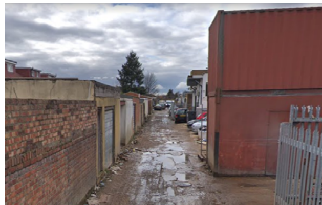
Examples of the environment along a typical service yard. Photos © Allies and Morrison
