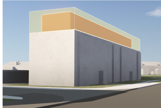
2 The upward extension is set back to preserve the street profile and to distinguish new and old. The massing and height is subordinate to the existing buildings.
