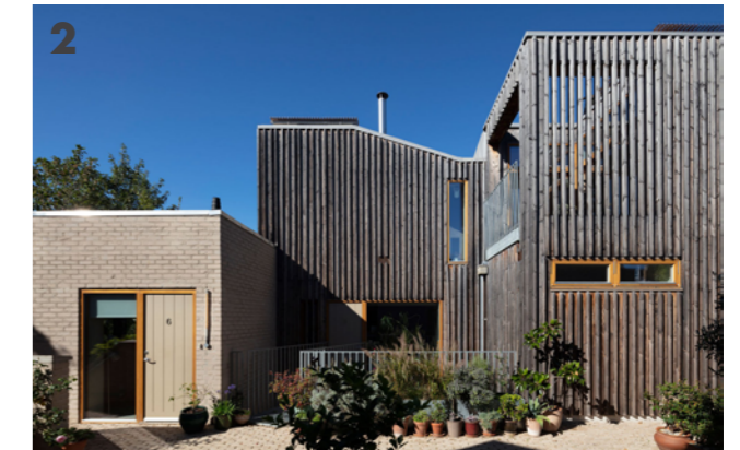
1 Garden House by Hayhurst & Co © Kilian O'Sullivan - Three different roof pitches respond to the scale of the neighbouring buildings. Stepped trays on the roof provide level planting beds which the occupants can actively garden.
