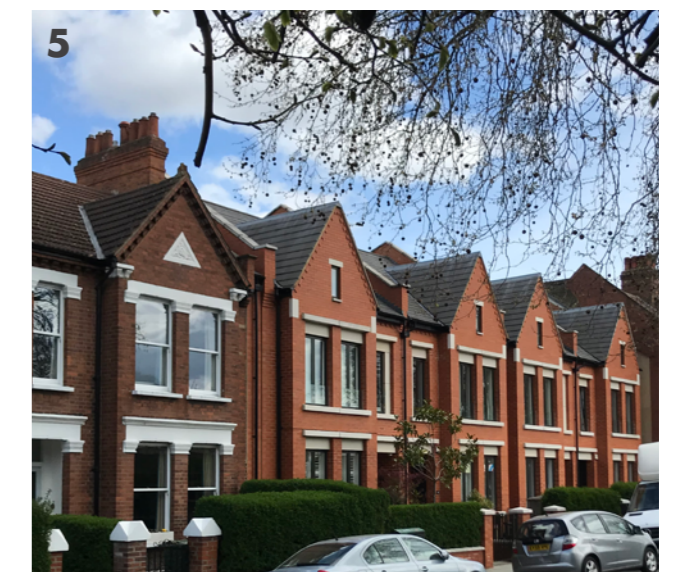
5 14 - 17 Calais street, Camberwell, Private developer - Four home residential infill development in a historic conservation area. © Allies and Morrison
