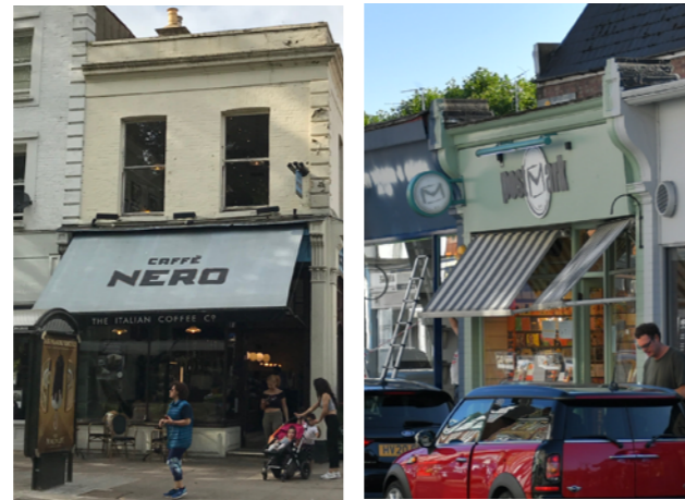
Fig A2.50 Appropriate canopies, 386 Chiswick High Road (left) and 53 Turnham Green Terrace (right). Photo credit: ©Allies and Morrison
