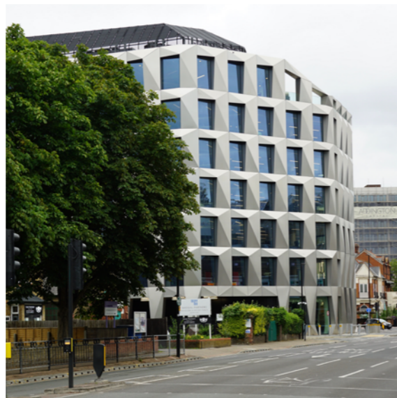
Fig A2.14 Civic buildings such as the new Council offices in Hounslow should be landmark features in the townscape. © Allies and Morrison
