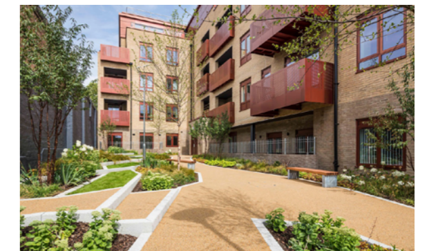
Fig A2.11 Church Road, Leyton apartments heated through a large scale air source heat pump which feeds a communal ambient heat network © Osel Architecture
