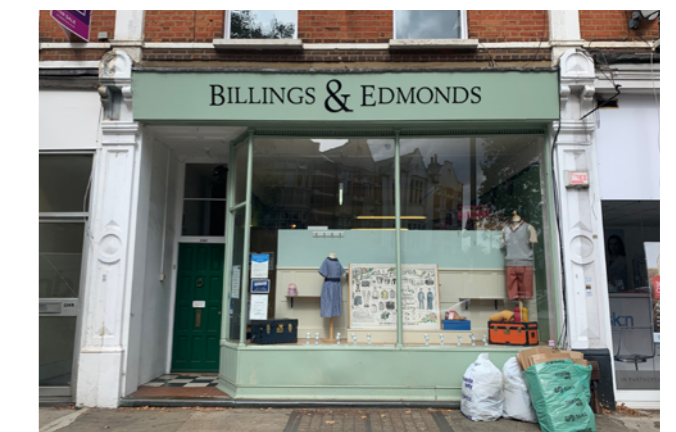
Fig A2.49 Well proportioned shop front and fascia, retaining original door arrangement, 112 Chiswick High Road.
