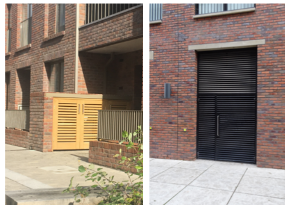
Fig A2.26 Examples of waste and recycling storage integrated into the overall built form of the development. © Allies and Morrison
