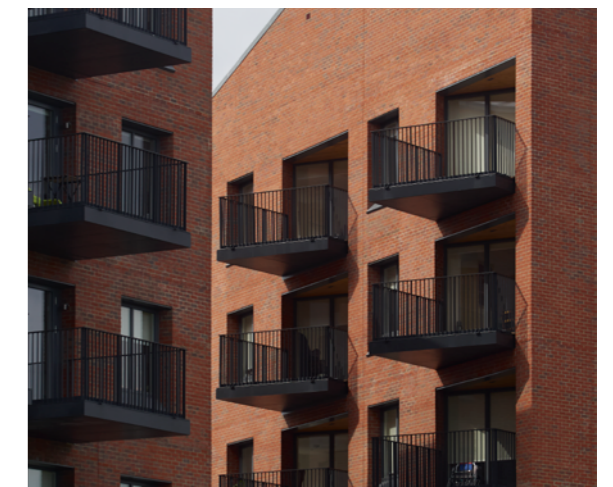
Fig A2.40 Semi inset and protruding balconies provide privacy and shelter for residents. Lock Keepers, Bow by Allies and Morrison architects. Photo credit: © Nick Guttridge
