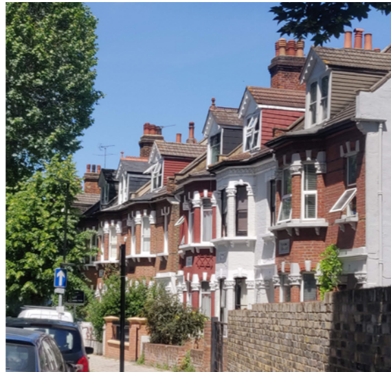
Fig A2.13 Many of the borough's residential streets demonstrate how the attention to detail and the use high quality materials can support a strong and enduring identity. © Allies and Morrison
