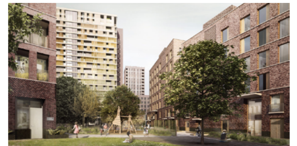
Fig A4.12 Agar Grove is a high density mid/high-rise Passivhaus development promoting a 'fabric-first' approach to energy performance and human comfort ©Hawkins/Brown
