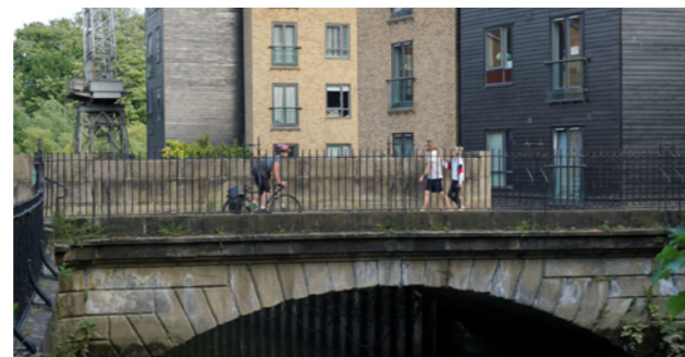
Old Isleworth's Riverside Mill (Manor House Way) takes cues from its riverside setting and industrial uses formerly on site
