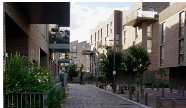
Brentford Lock West (by Duggan Morris) is an award-winning example of contemporary development which carries through historic threads of the canalside context in its design
