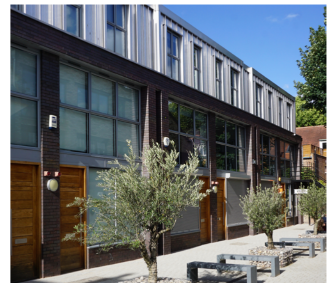
Turnham Green Terrace Mews is an example of backland intensification, now providing workspace, food and retail
