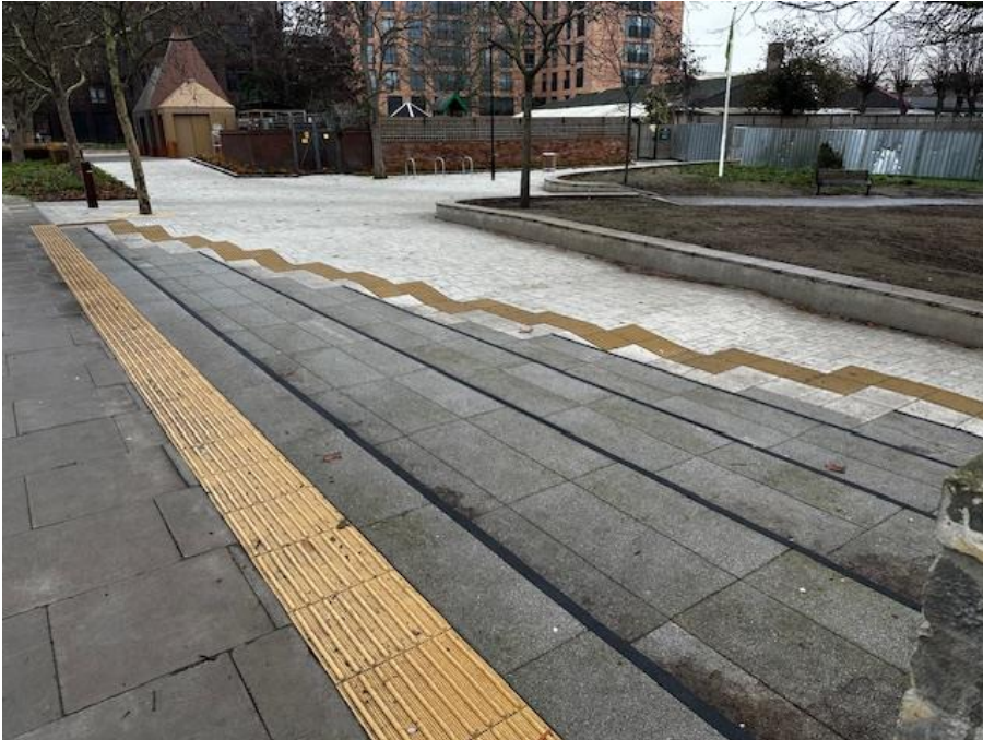
Figure 3 New granite steps leading into the new memorial and cabin area
