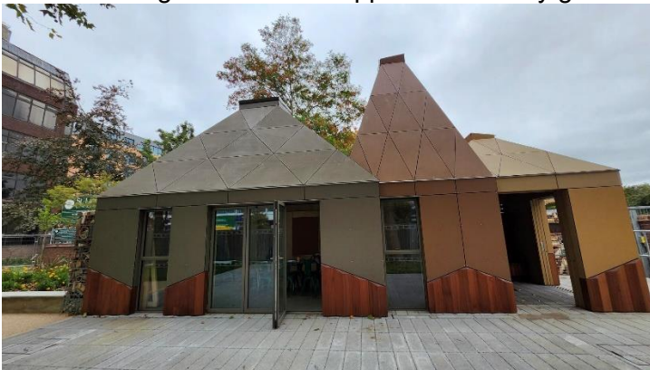
Figure 22 Completed Eco Cabin
