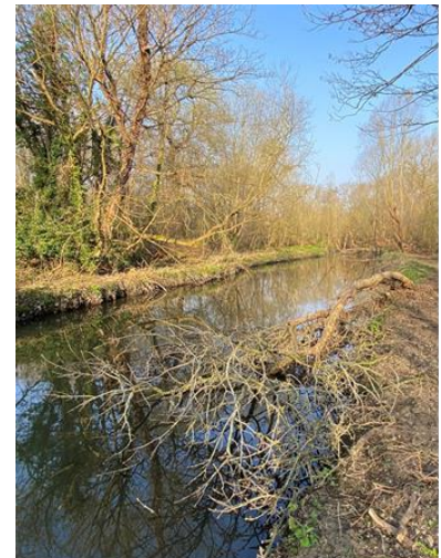
Tree flow deflector installed at Little Park, March 2022
