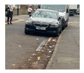
The extent of the road markings introduced also does not accord with the design drawings presented for audit. This has resulted in indiscriminate parking along this section of the carriageway. Indiscriminate parking causing obstruction to the carriageway which may increase the risk of pedestrian strike and/or result in reversing or avoidance manoeuvres and potential for sudden braking and rear end shunts with other road users.
