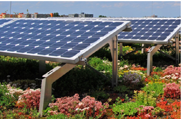
Figure 3.5 – Combining Solar PV panels with green roof systems
