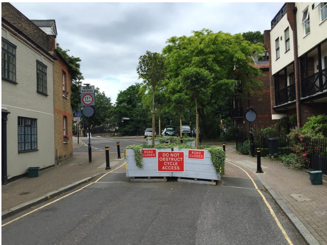
Figure 1.1: Church Street Closure
