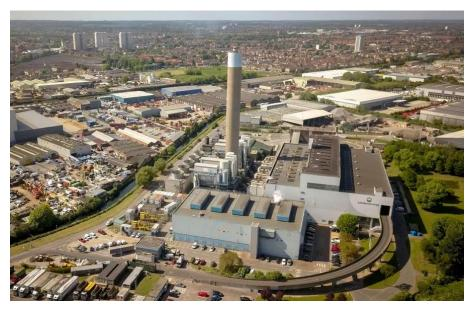
Figure 4.7 - Energy from Waste heat networks are centred around using heat that is produced by the process of waste incineration (above the North London Edmonton incinerator) distributing that heat to homes close to it or much further (Photograph: pxl.store/Alamy)
