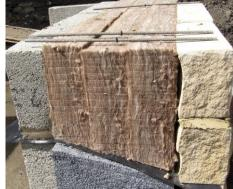
Figure 11.15 - Good examples of insulation installed on site, showing methods to eliminate gaps (wedging and overfilling). Left: Goldsmith street © Etude, Right: © Green building store.
