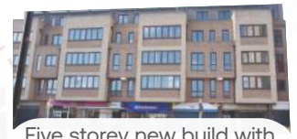
Five storey new build with residential on top of retail units
