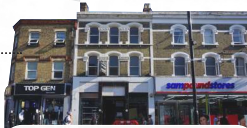
3 Storeys 1900 stock brick, terracotta ornament, stone lintels with stop moulds, and Italianate mouldings
