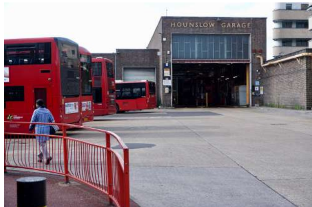
Figure 1.50: Photos of the existing bus garage
