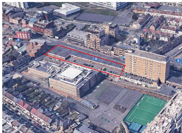
Aerial view of existing area
