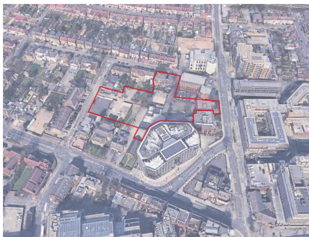
Aerial view of existing area
