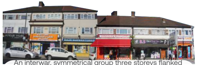
An interwar, symmetrical group three storeys flanked by two storey wings. Retail with perhaps residential units above. Much of these buildings have been altered, though one Crittall window remains.
