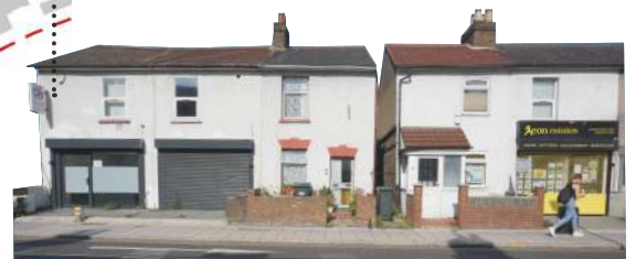
Two storey late 19th century cottage style terraces, mostly retail, and heavily altered - including doors, windows, roofs, and boundary walls.
