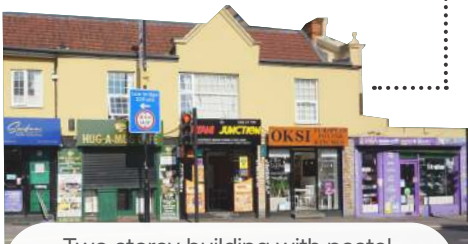
Two storey building with pastel yellow render, and gables with much of it altered. It was Formerly the Duke of Wellington public house.
