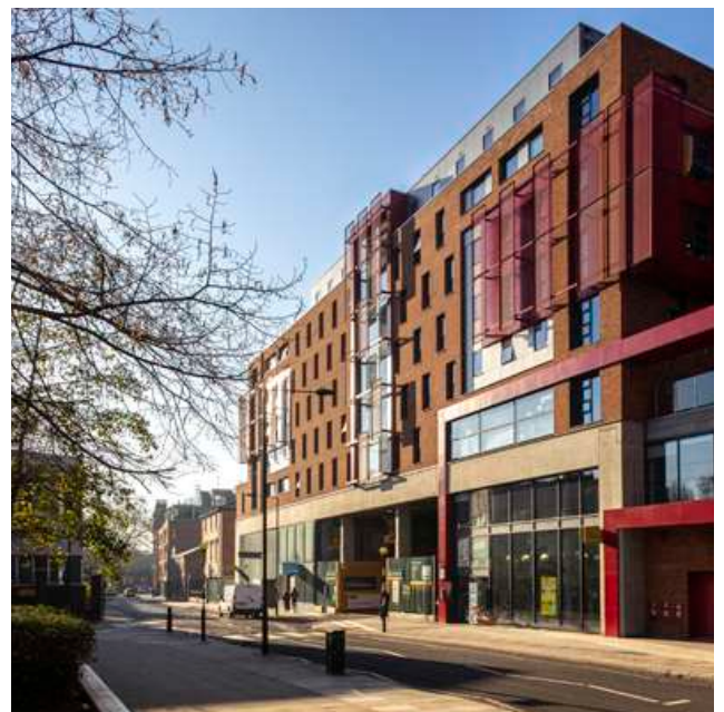
Unite and Travis Perkins © Cooley Architects
