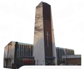
1961 Church by W E Cross. Concrete obelisk tower
