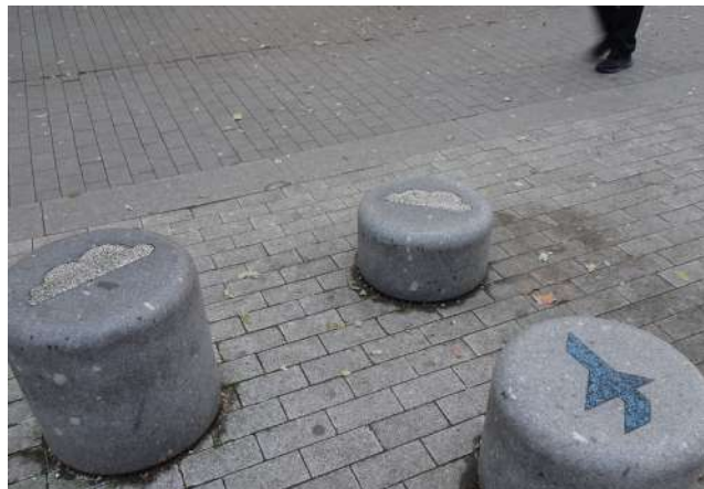
Hounslow town centre lacks greenery which would soften the urban environment and bring greater climate resilience. The grey low bollards are particularly difficult to see, and as such are a barrier to accessibility.
