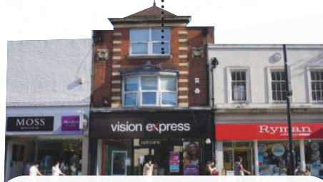
1920s Georgian revival, red brick canted first floor window, stone garlands, cornice and hipped roof
