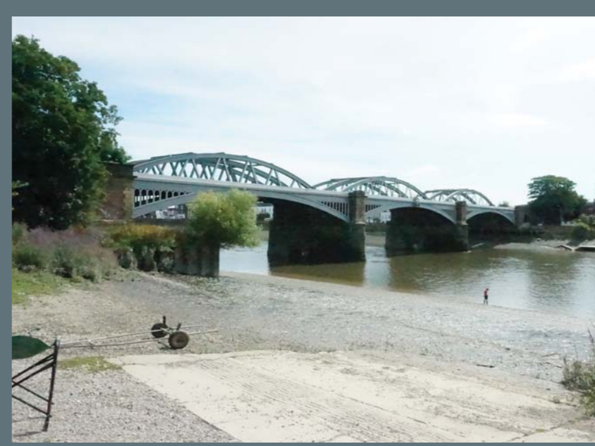
Pedestrian Bridge and slipway
