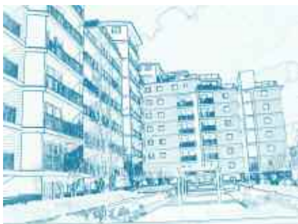
New Housing Development, Brentford
