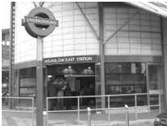
Hounslow East Underground Station
